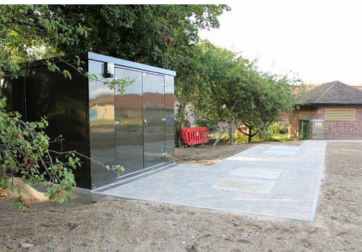
A recent PWS installation where only the kiosk is visible above ground, the tanks having been buried.
